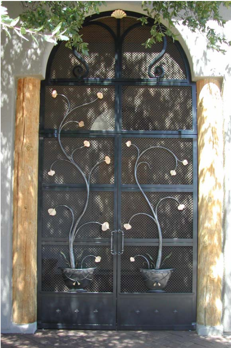
"Vine of Life" screen doors, 12'6" tall and 6" wide, are mounted on 2-speed, in-ground automatic closers with hold open feature.
