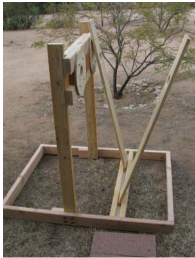
Photo 3. Frame for the double bellows under construction..
