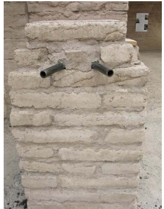
Photo 7: Fabricated black pipe Y-fitting/tuyere embedded in adobe mortar in the forge.
